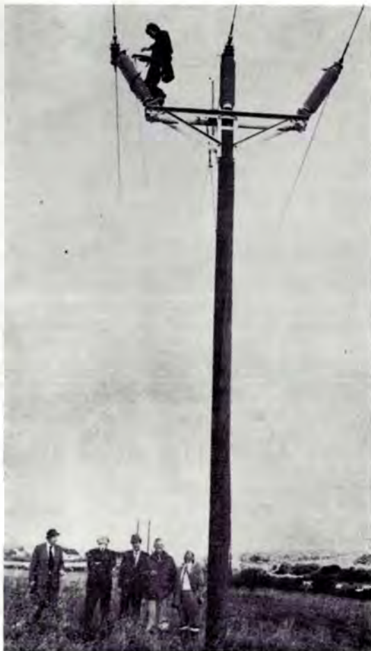
Inside a safety rope enclosure, the linesman demonstrates the ease of working on the line end of one of the outside insulators. Below, without crash helmets as this was a posed-for picture, are Messrs. Mike Hughes, Arthur Perry (Asst. Chief Engineer, Construction), Des Wallin (Murphy's), Ken Jones and Geoff Price.
